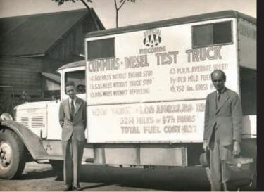
In 1931, a Cummins-powered truck demonstrated reliability and fuel efficiency in a cross-country run from New York to Los Angeles, averaging 33.03 mph and beating the record held by General Motors, with a running time of 97 hours, 20 minutes. The truck averaged 15.75 mpg, and fuel for the 3,214-mile trip cost \$11.22.
